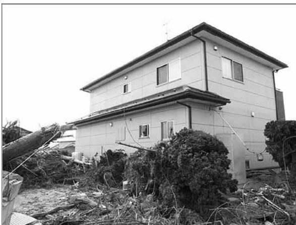
P7.A House Which Withstood the Attack of 2011 Tohoku Earthquake and Tsunami (3)
